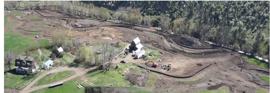
Catherine Creek, RM 44, Southern Cross Conservation Property Fish Habitat Restoration
